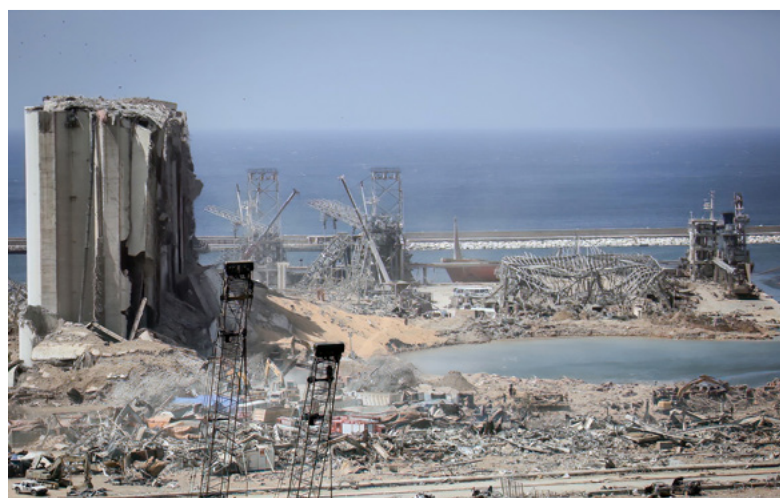
Damage after the Beirut explosion, Mehr News Agency, CC BY 4.0
